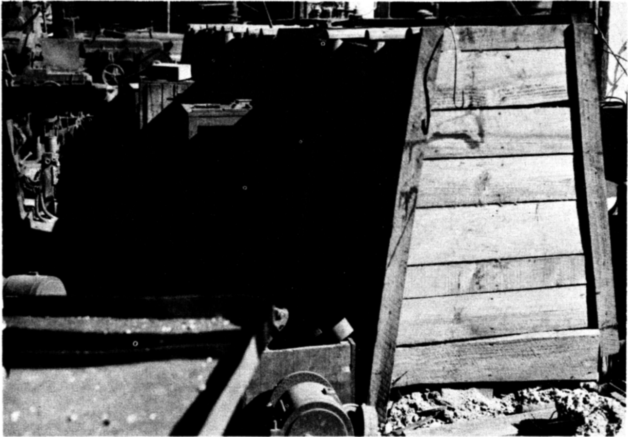
Figure 12.37c. Earth-filled, wooden blast walls protecting machinery (0.85 mile from ground zero at Nagasaki).
